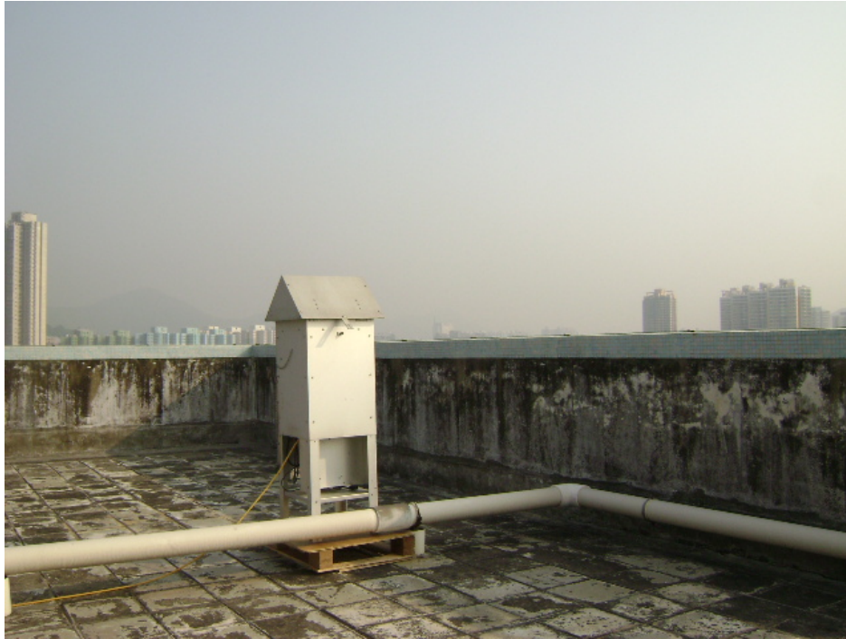
Roof top of Block 15, Yuet Wu Villa
