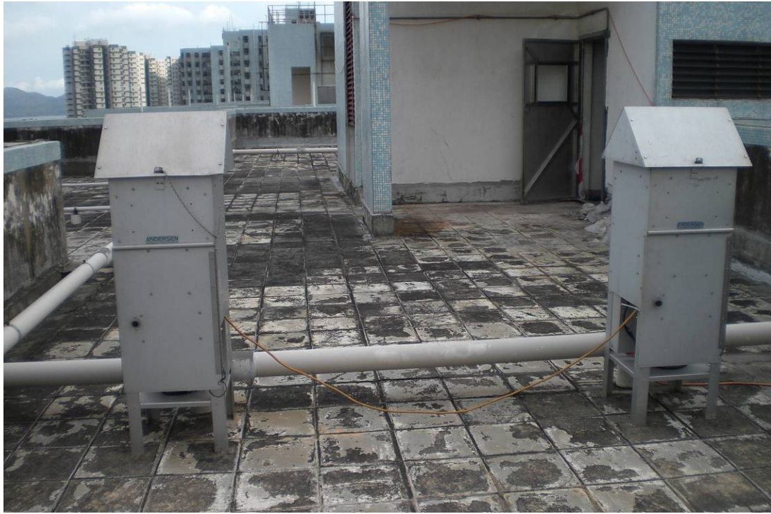
Roof top of Block 15, Yuet Wu Villa
