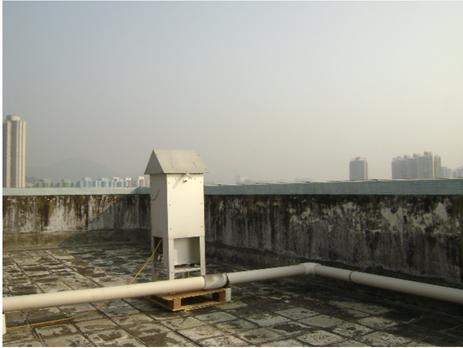
Roof top of Block 15, Yuet Wu Villa
