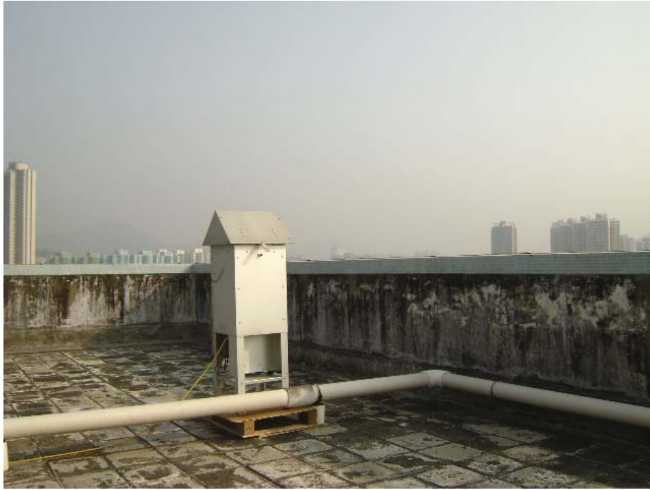
Roof top of Block 15, Yuet Wu Villa
