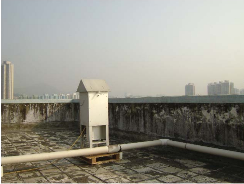
Roof top of Block 15, Yuet Wu Villa
