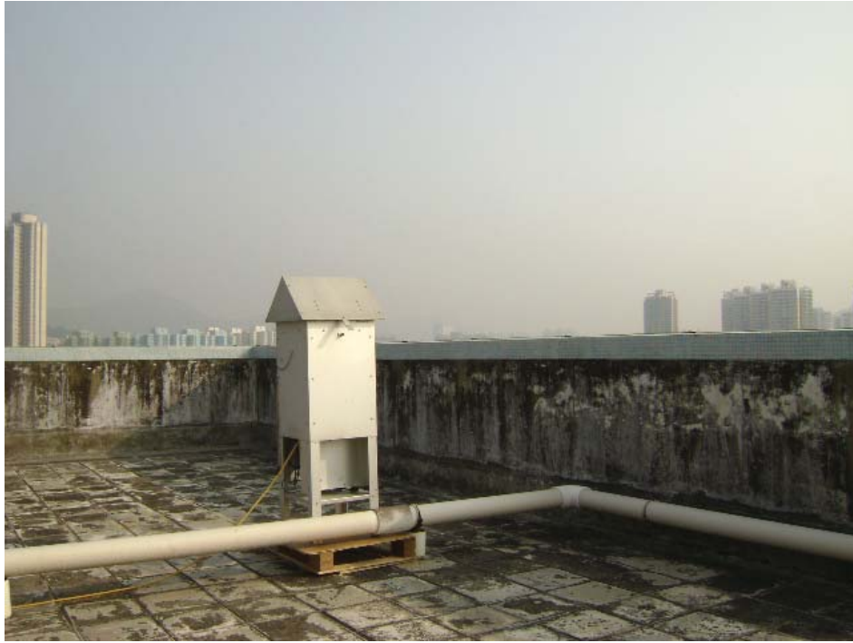
Roof top of Block 15, Yuet Wu Villa
