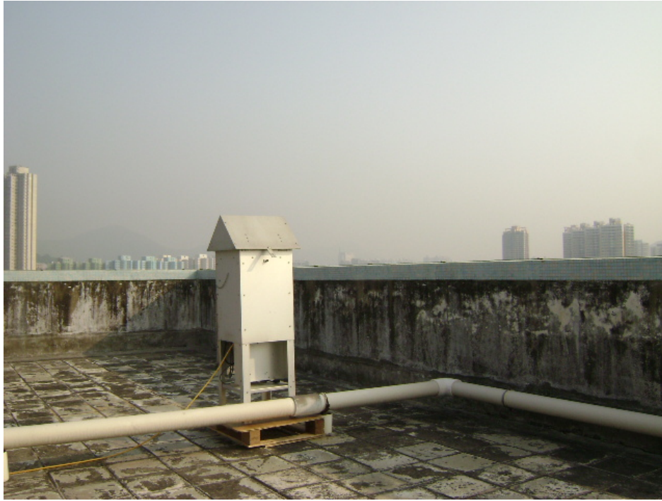
Roof top of Block 15, Yuet Wu Villa
