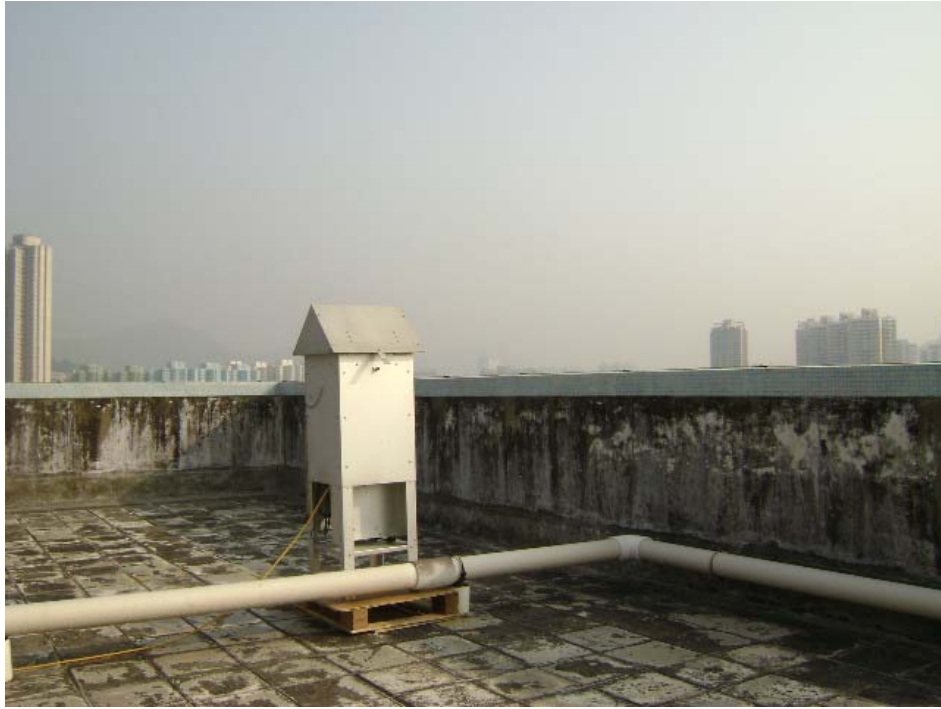
Roof top of Block 15, Yuet Wu Villa
