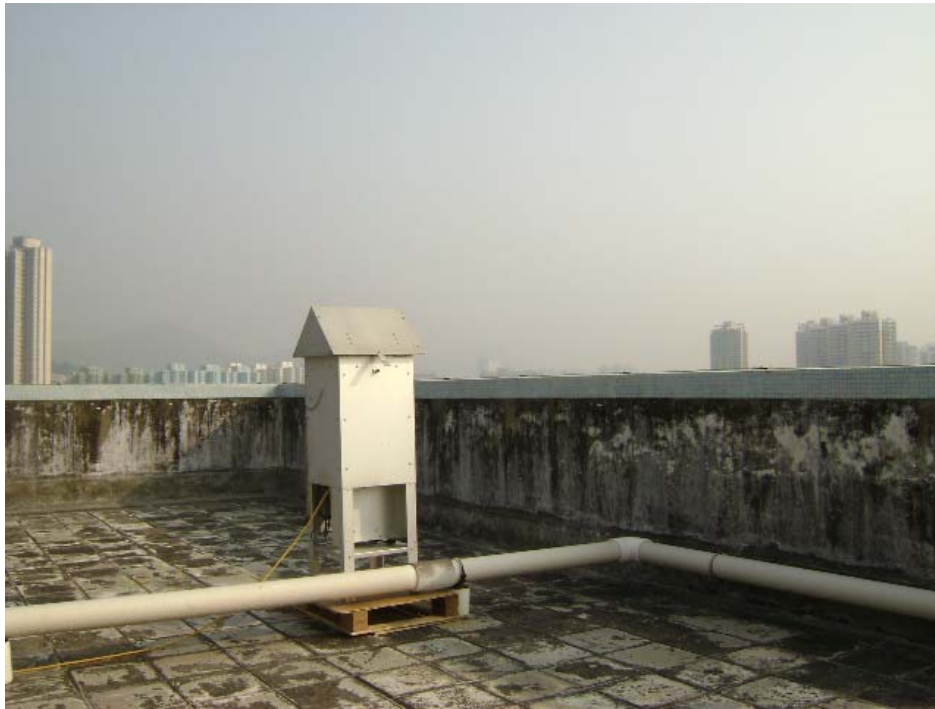
Roof top of Block 15, Yuet Wu Villa
