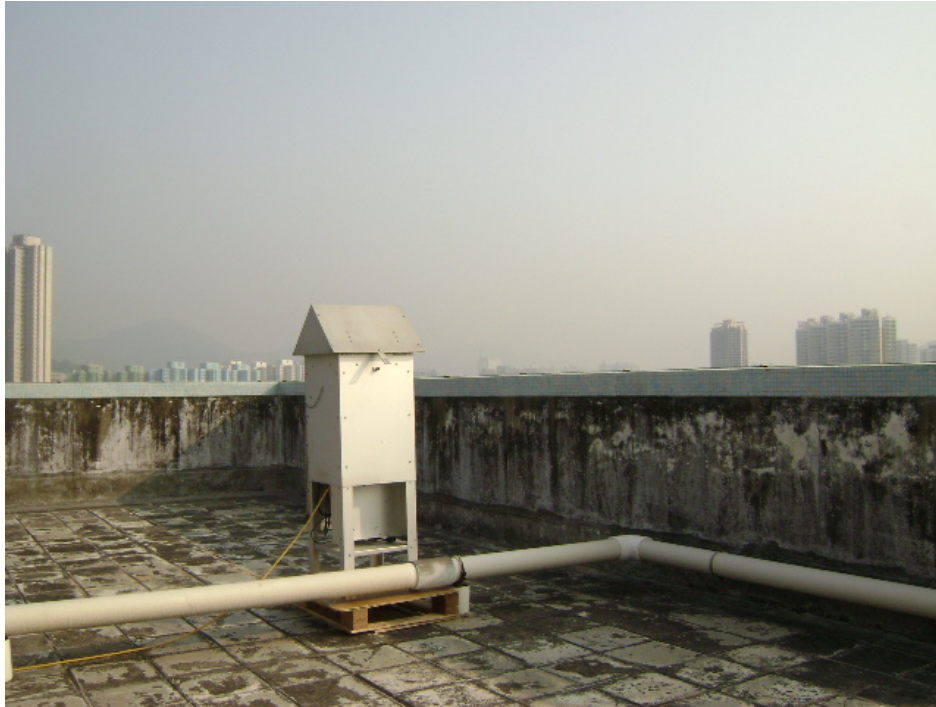
Roof top of Block 15, Yuet Wu Villa
